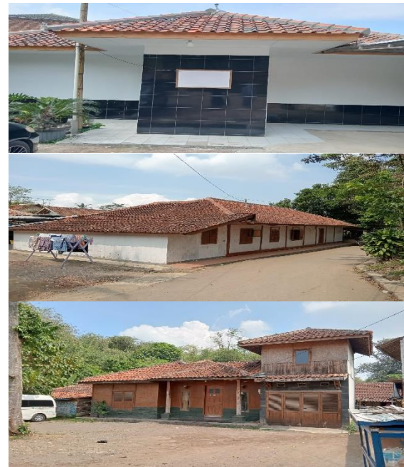
Source: Researcher's Document, 2024 Figure 1. A building made of brick and glass in Kampung Mahmud
