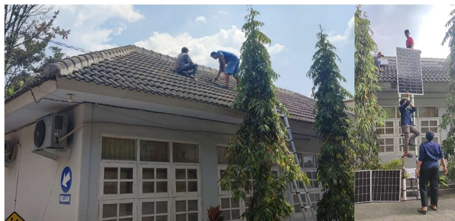
Gambar 3. Proses Instalasi Panel Surya
