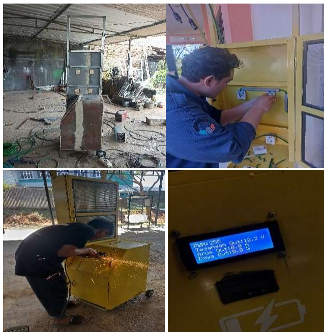
Gambar 3. Pembangunan Teknologi Solar Electric Device Charging Station
